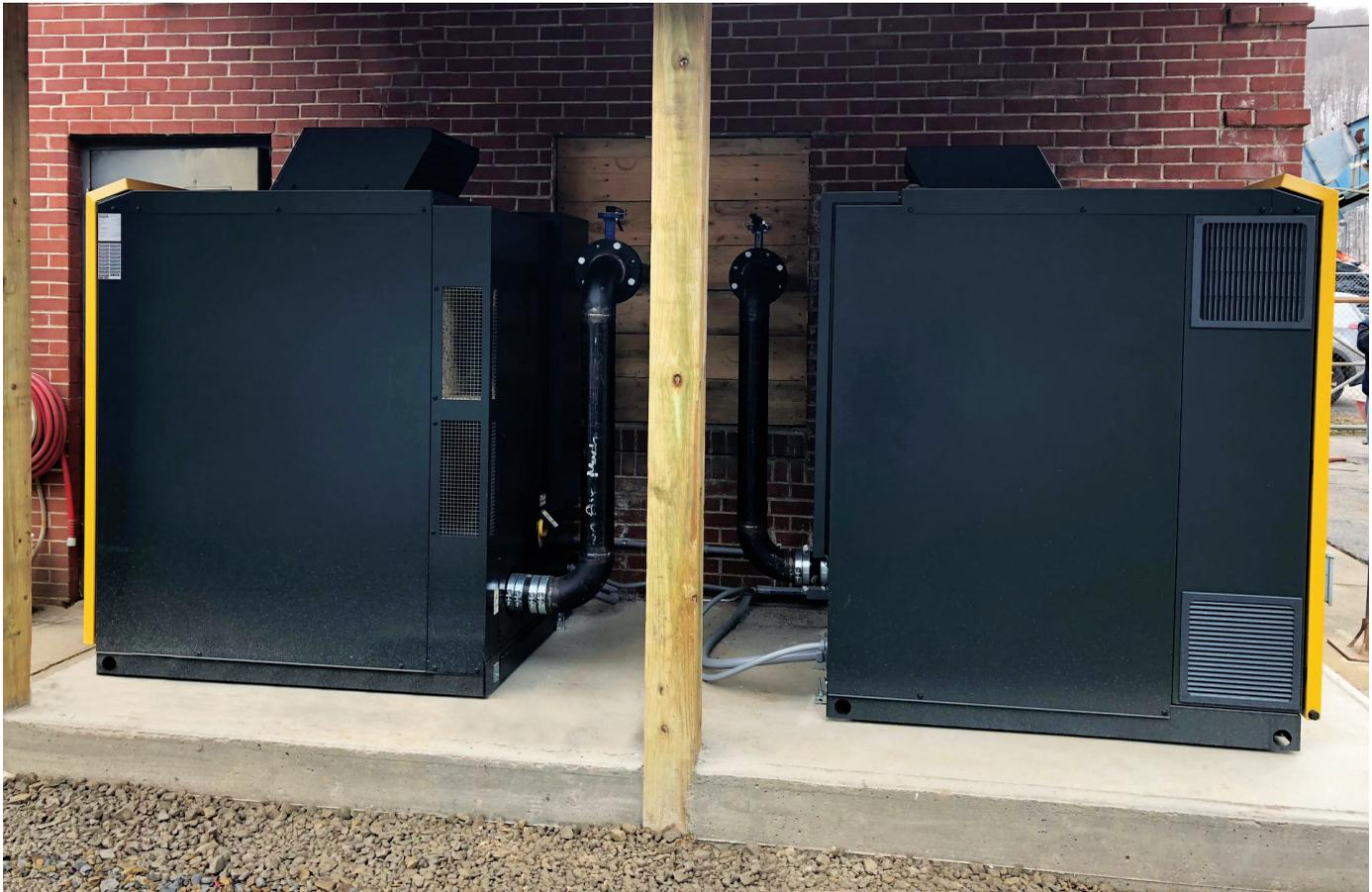
DBS screw blowers with variable frequency drives helped Chapmanville Water Department lower its energy expenses while also upgrading its failing blowers.
