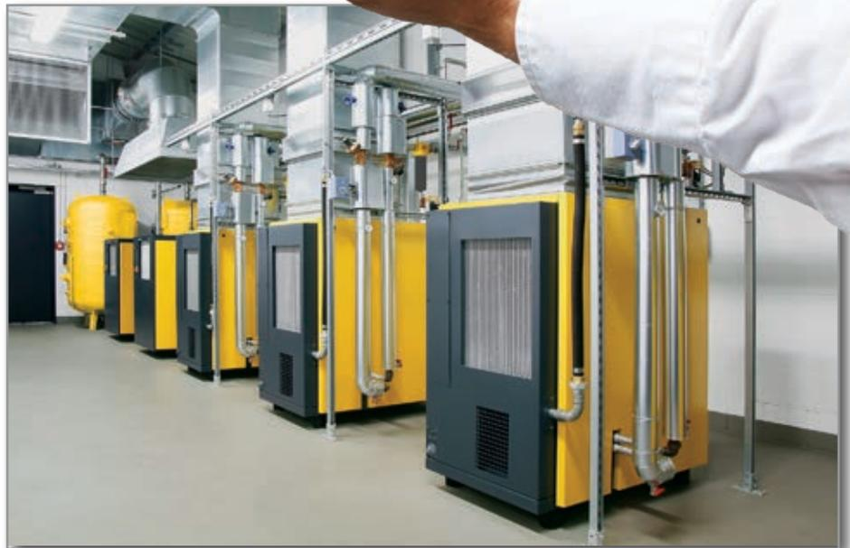
*Air-cooled, fluid-injected screw compressors with internal heat exchangers and controls to tap into the thermal energy of the cooling fluid. The additional ducting removes the hot air that was not rejected by the hot water recovery system.*
